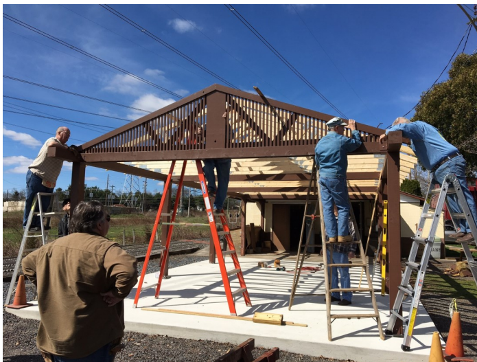
Final decorative truss is installed at the end of the pavilion
