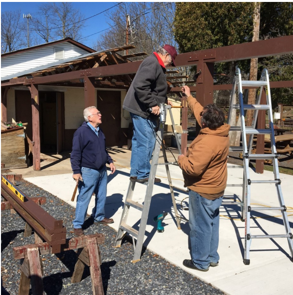
Bob Hillenbrand fastens metal "T" plates to posts and cross beams
