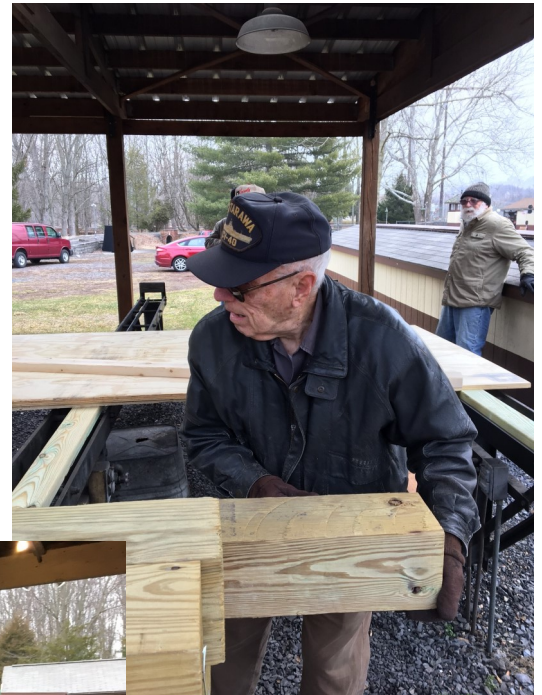
Walt Mensch stacks new lumber for the pavilion
