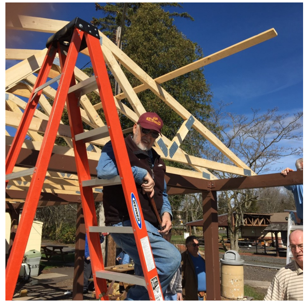
Bob Hillenbrand helps secure the trusses
