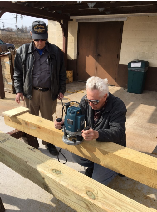
Frank Webb cuts chamfer for posts
