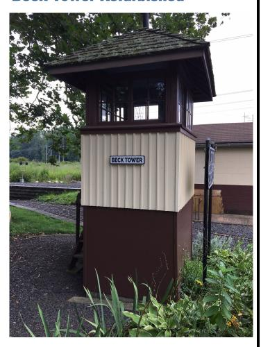
Refurbishing of the Beck Signal Tower was completed this past summer. The rotted outside wood trim was replaced with PVC and the railing and stairs were repaired with help from Ron Shupard. Most of the windows were re-glazed and the entire exterior was completely repainted. Also a new sign was added to replace the original which had fallen into disrepair years ago.
