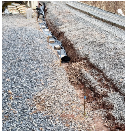
Photo 1 - Trench/Footing ready for New Wall
