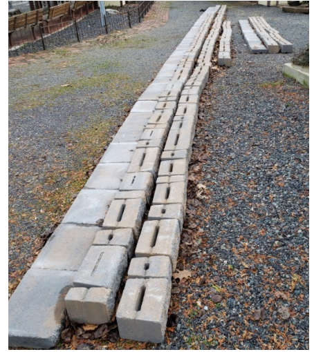
Photo 2 - Block Layout ready for transfer
