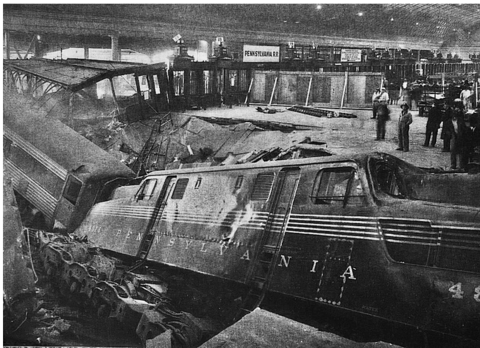
4876 rests on Baggage Room floor after crashing down from track level above.
