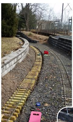
We finally got to the root of the problem. During the winter we pulled up 90 feet of track of the lead coming out of the 7 1/4" yard past the lower steaming bays. A lot of stone was removed and finally we got to the roots that were pushing the track out of shape. A tremendous amount of work was needed to remove these
