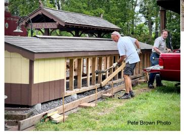
Rick and Terry frame up the supports for the ballast under the "Dog House" used to store the Company Train and Work Train.
