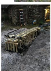
wide x 1/4" thick x 12' which gave me enough to make two stringers. After cutting, I layered them up in glue and clamped them in a curved jig till dry. Once dry, I was able to run them thru my planner to square them up and clean off any unwanted glue. Following that I spaced out the trestles over the stringers and fastened with stainless steel wood deck screws. I then assembled a section of curved track and fastened to the stringers.
