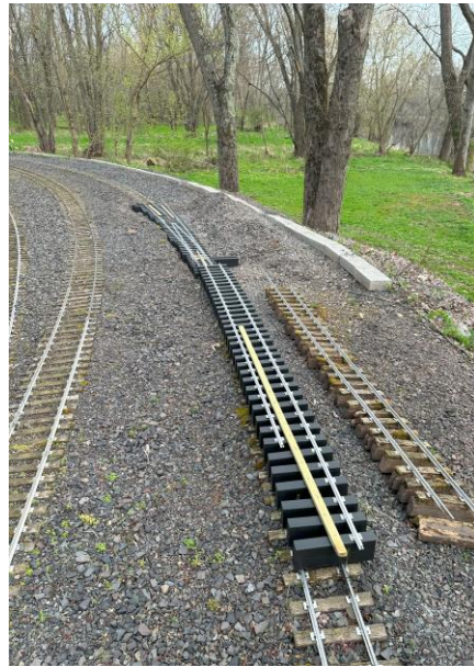
The new turnout at Mercer Bridge is in place and still needs to be connected to the 4.75 Main Line on both ends.
