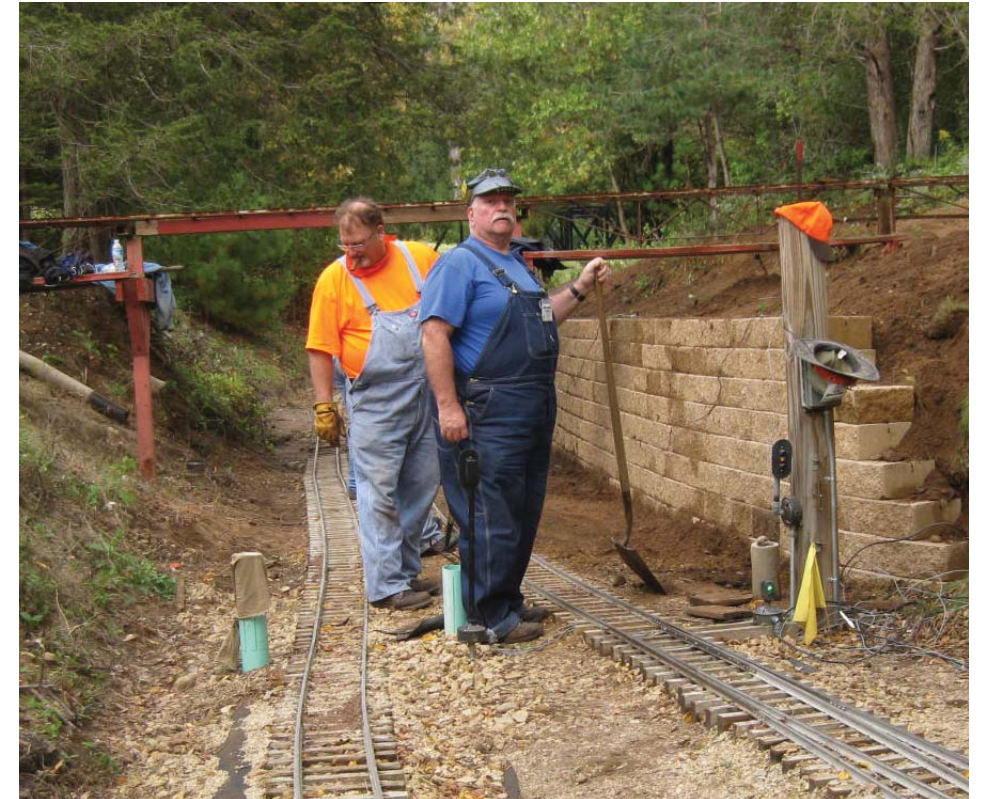
John Bortz helps set a retaining wall built of 82 pound block.
