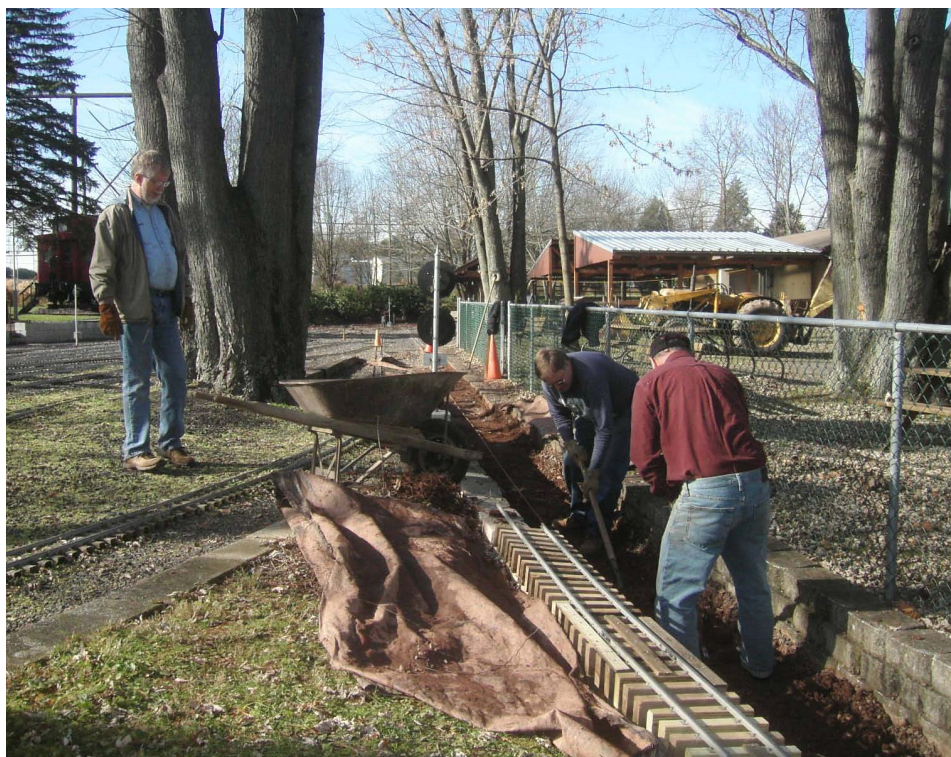
PLS Workers set new track section in the cut leading to the brick tunnel.
