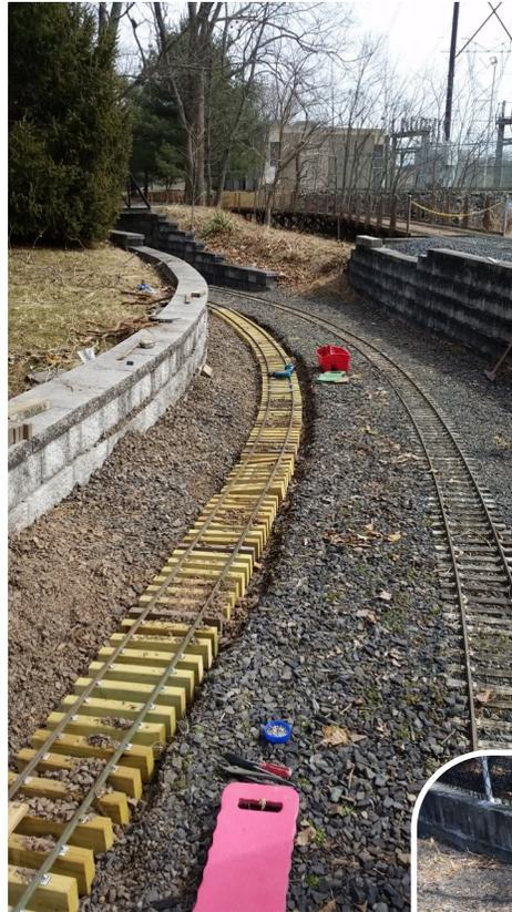
We finally got to the root of the problem. During the winter we pulled up 90 feet of track of the lead coming out of the 7 1/4" yard past the lower steaming bays. A lot of stone was removed and finally we got to the roots that were pushing the track out of shape. A tremendous amount of work was needed to remove these roots so we could put in the new track sections.
