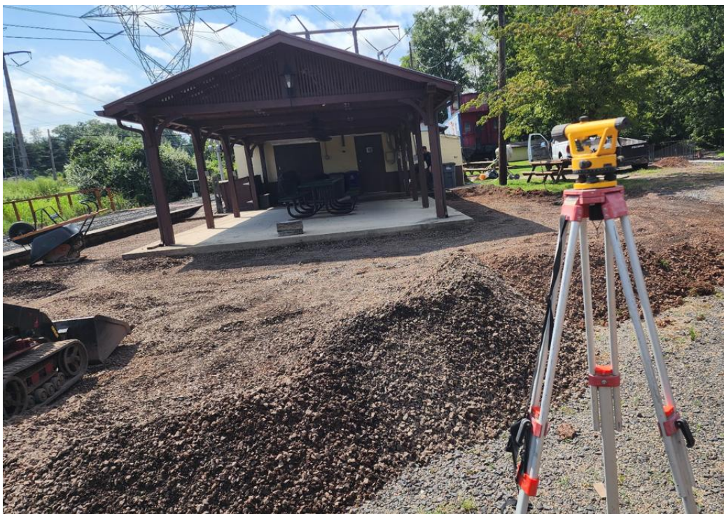
Paver Project off to a good start. Shown is the ongoing installation of the base layer. Photo by Steve Cortéal
